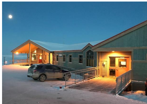
Nursing Station in Pond Inlet
